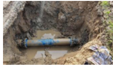
Repair to 200mm asbestos main, Arklow
