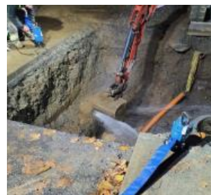
Repair to a leak on a water main, Bray
