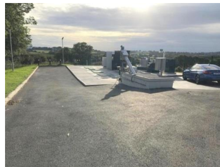
Ballyconnell Waste Water Treatment Plant
