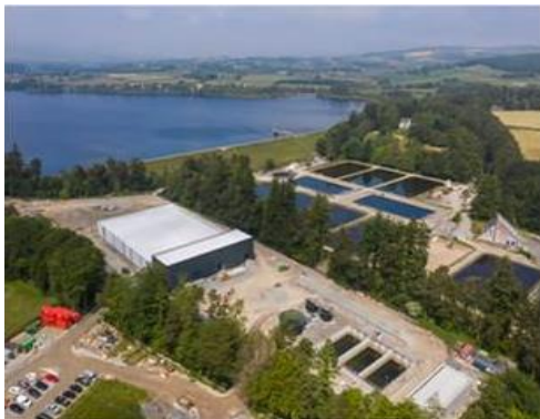
Aerial view of the Vartry Water Treatment Plant
