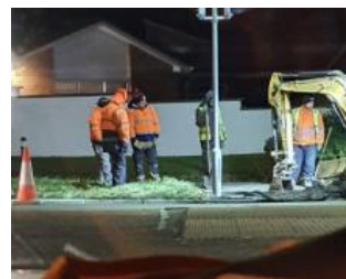
Repair to a leak, Mill Road, Greystones
